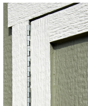
Figure 12.3 - Piano hinge
