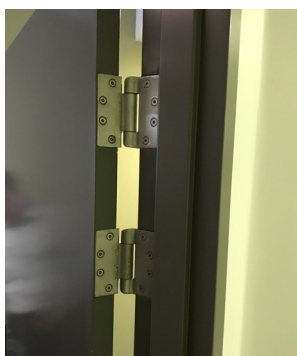
Figure 12.1 - Butt hinge
